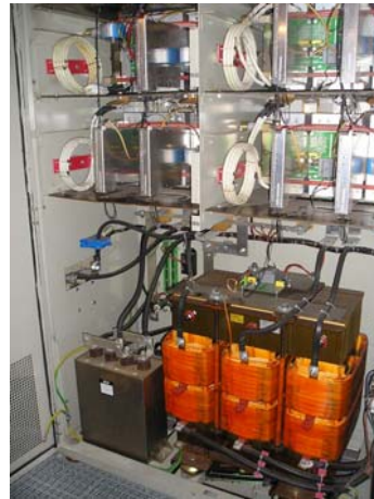
Detall armari convertors.
